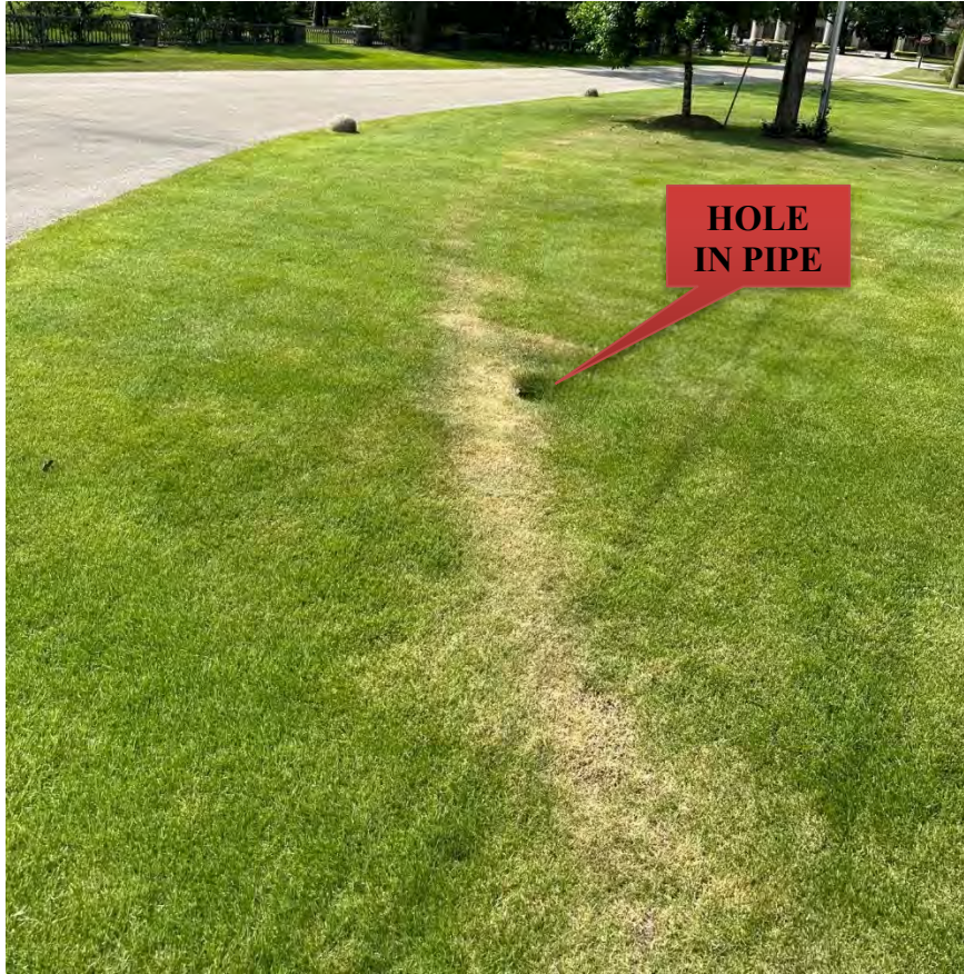
610 Grecian Way Storm Sewer
