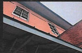
Gutters Unknown Custom Fab
