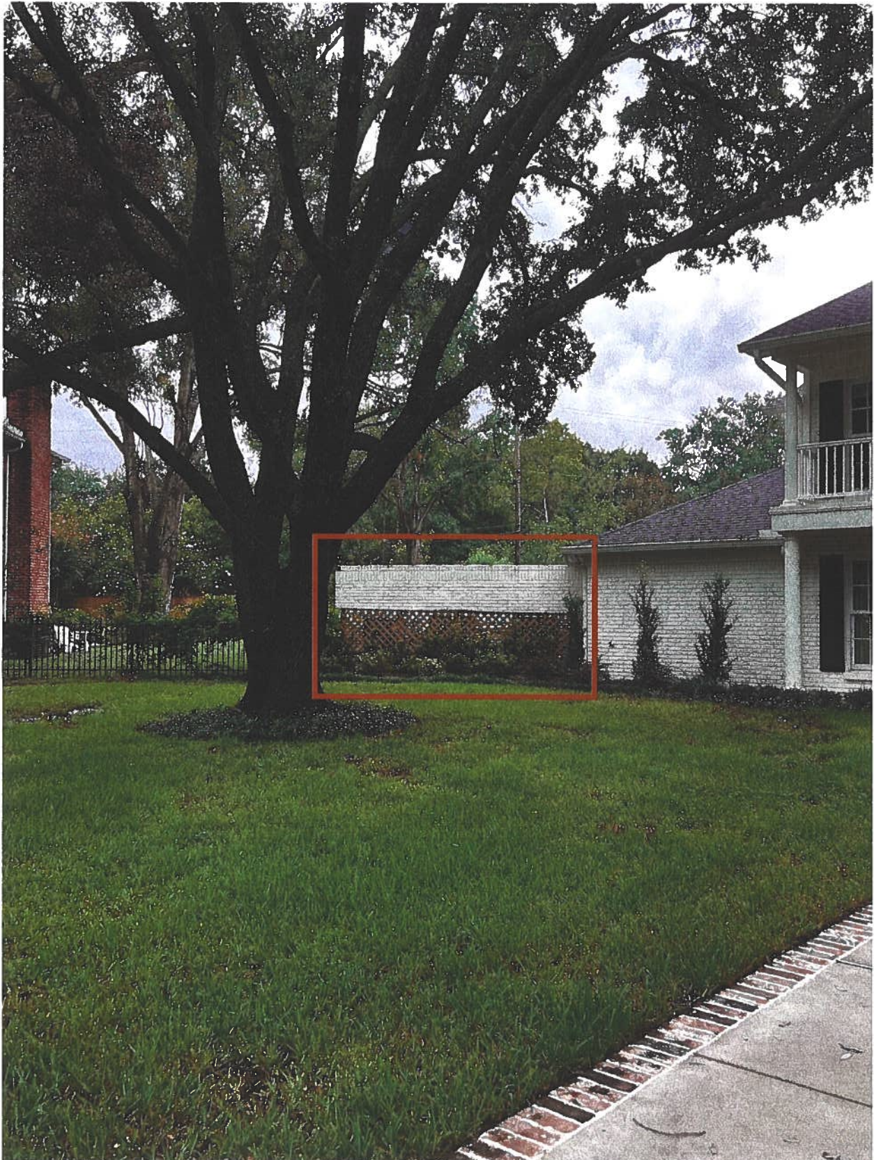
View of brick enclosure from street
