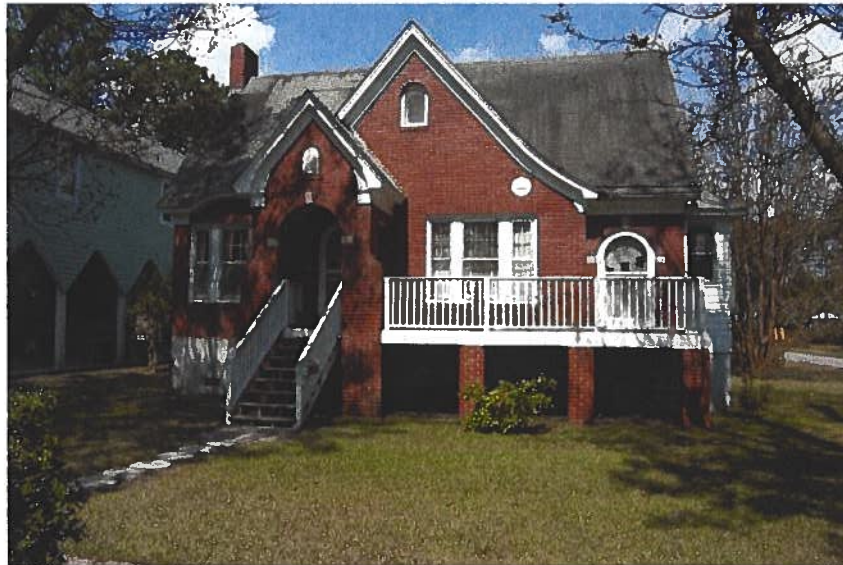
Frame building elevated on concrete block foundation faced with brick veneer. Belhaven, North Carolina.
