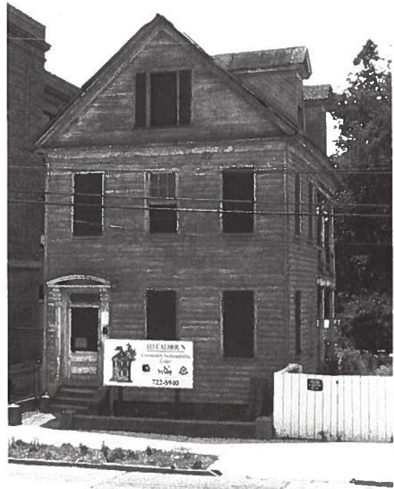
113 Calhoun at inception of project Photo courtesy of 113 Calhoun Street Foundation.
