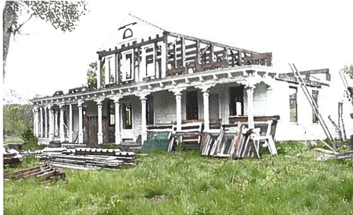
Dismantling of Bruchmann residence, May 2000
