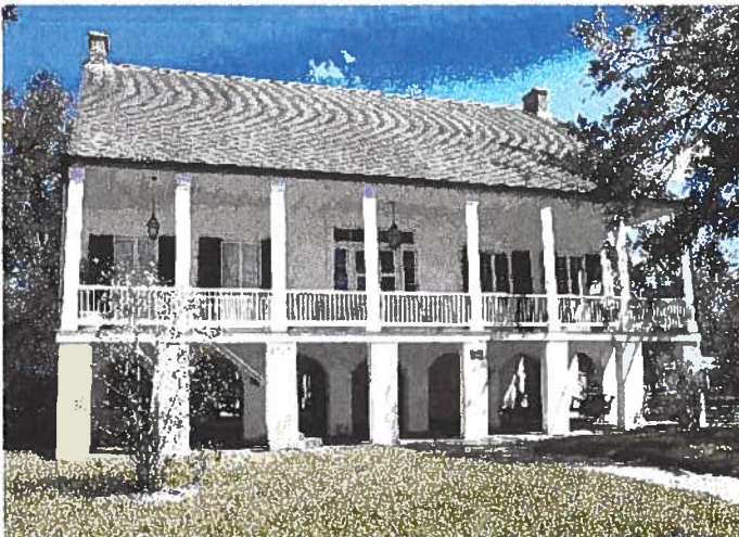
Elevation of a historic residence in Mandeville, Louisiana
