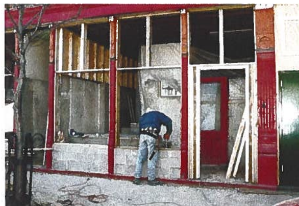
Floodproofing the vestibule of a storefront
