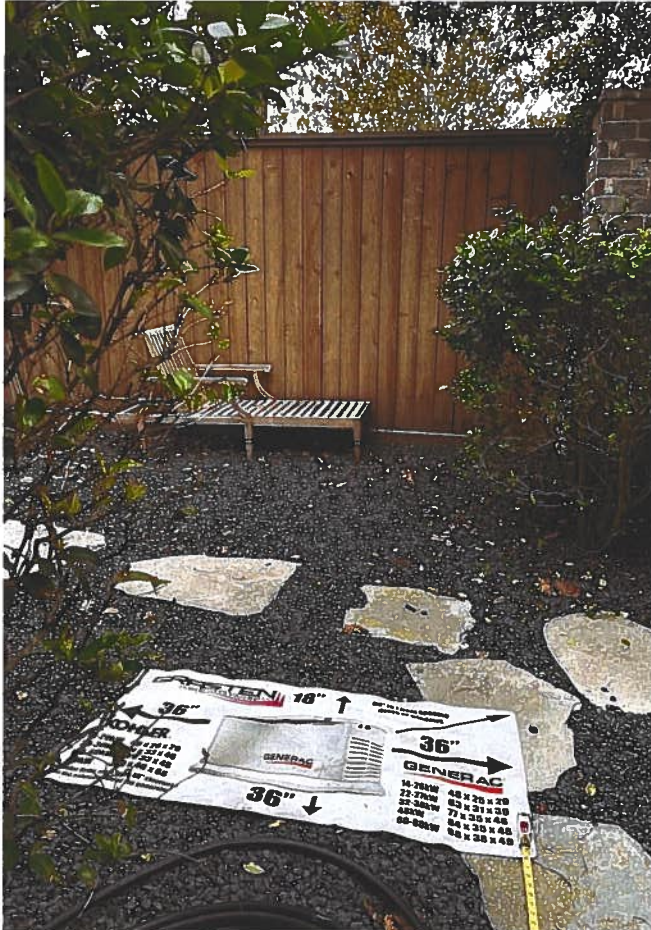
Exhibit C. Proposed location of generator – image looking east – 16.1' and 14.0' from the property line along the east side of our home.
