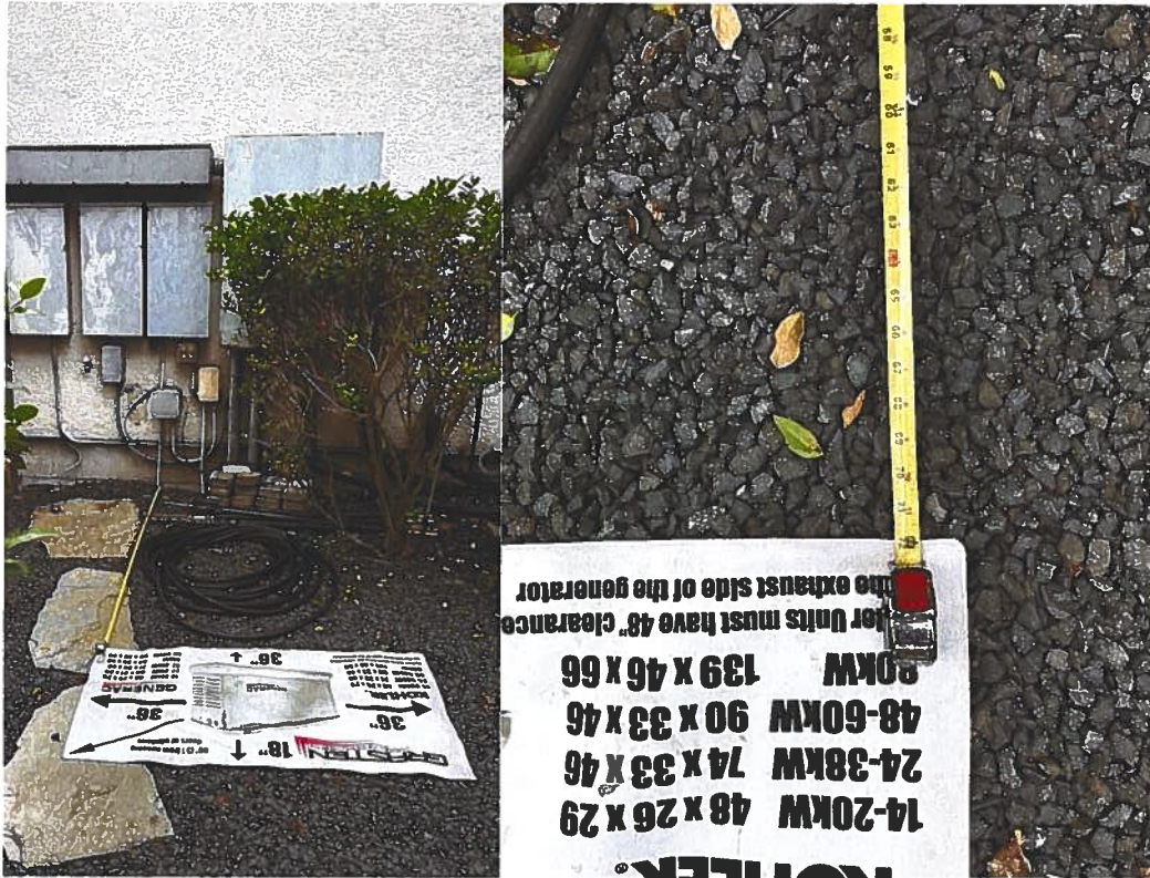
Exhibit D. Proposed location of generator – image looking west – 6' from the main structure along the east side of our home.
