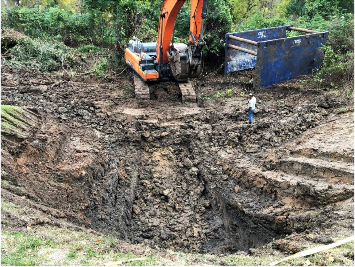
Sinkhole Excavation for Trench Box Installation 12-2-2022
