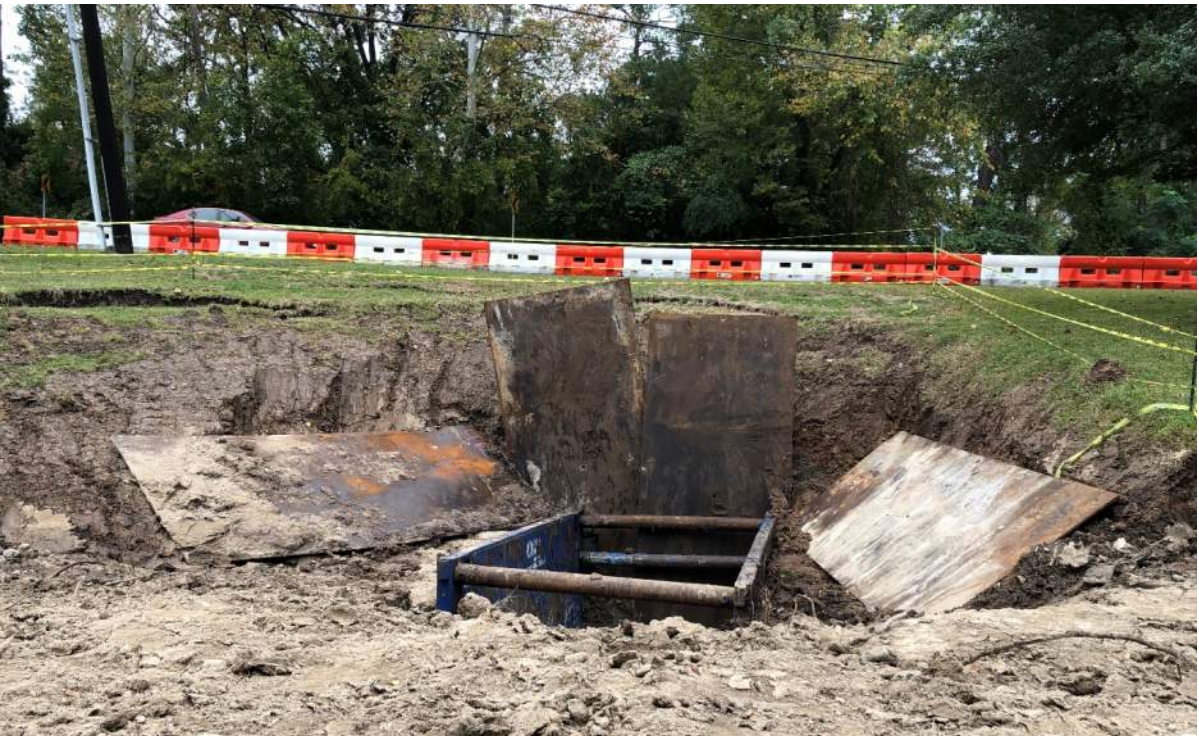
Sinkhole Excavation for Trench Box Installation 12-5-2022
