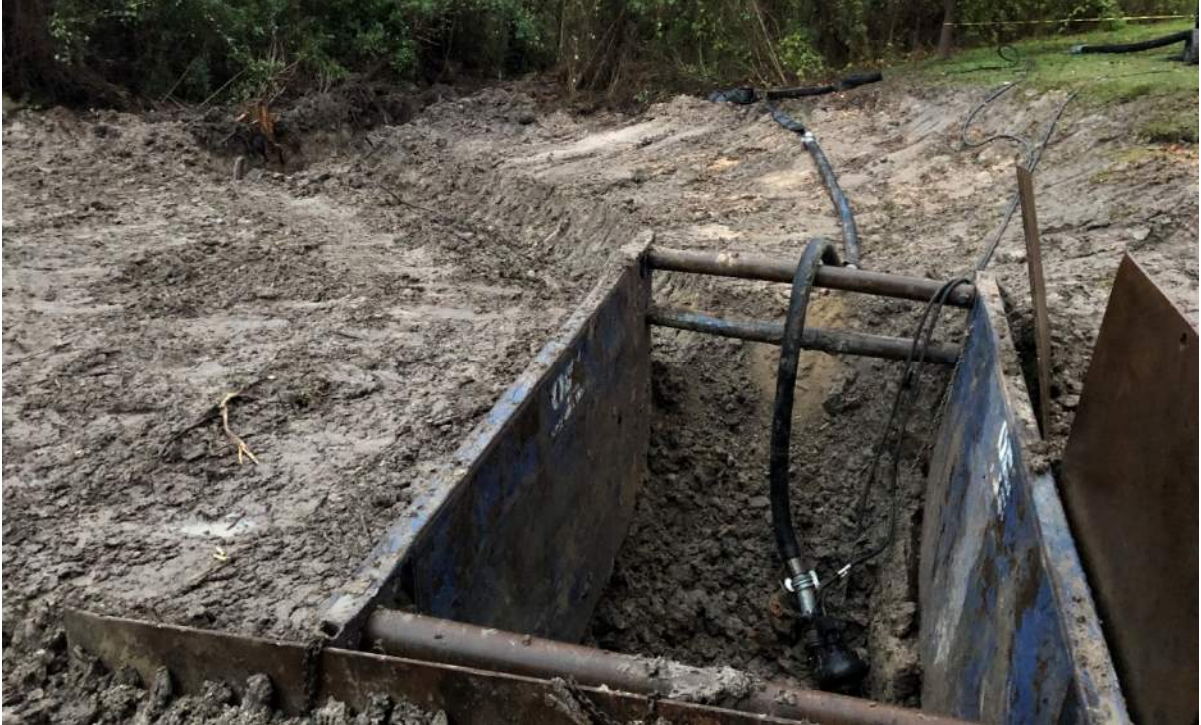
Site Preparation for Vac-Trucks 12-14-2022
