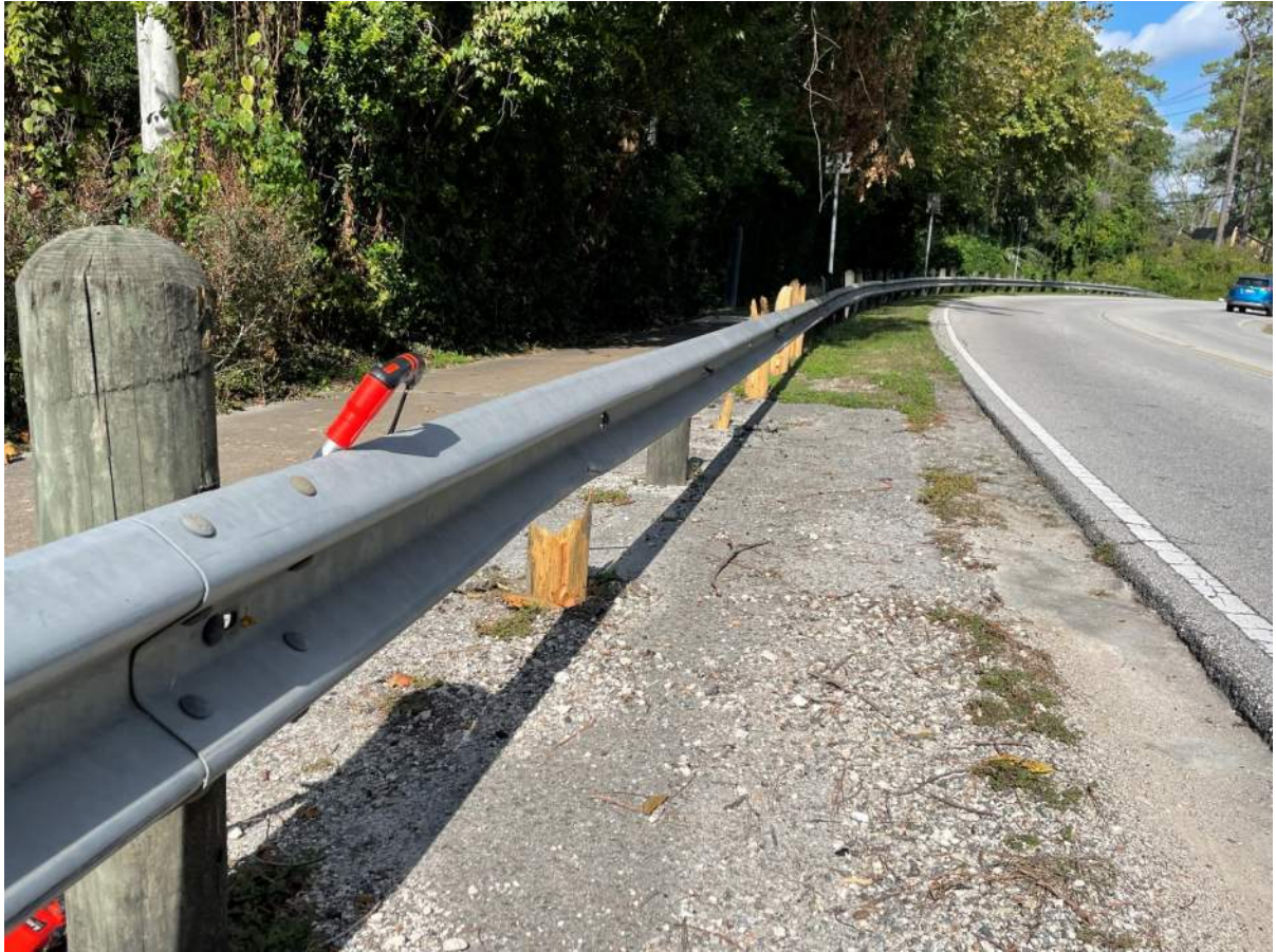
South Piney Point Road Guardrail
