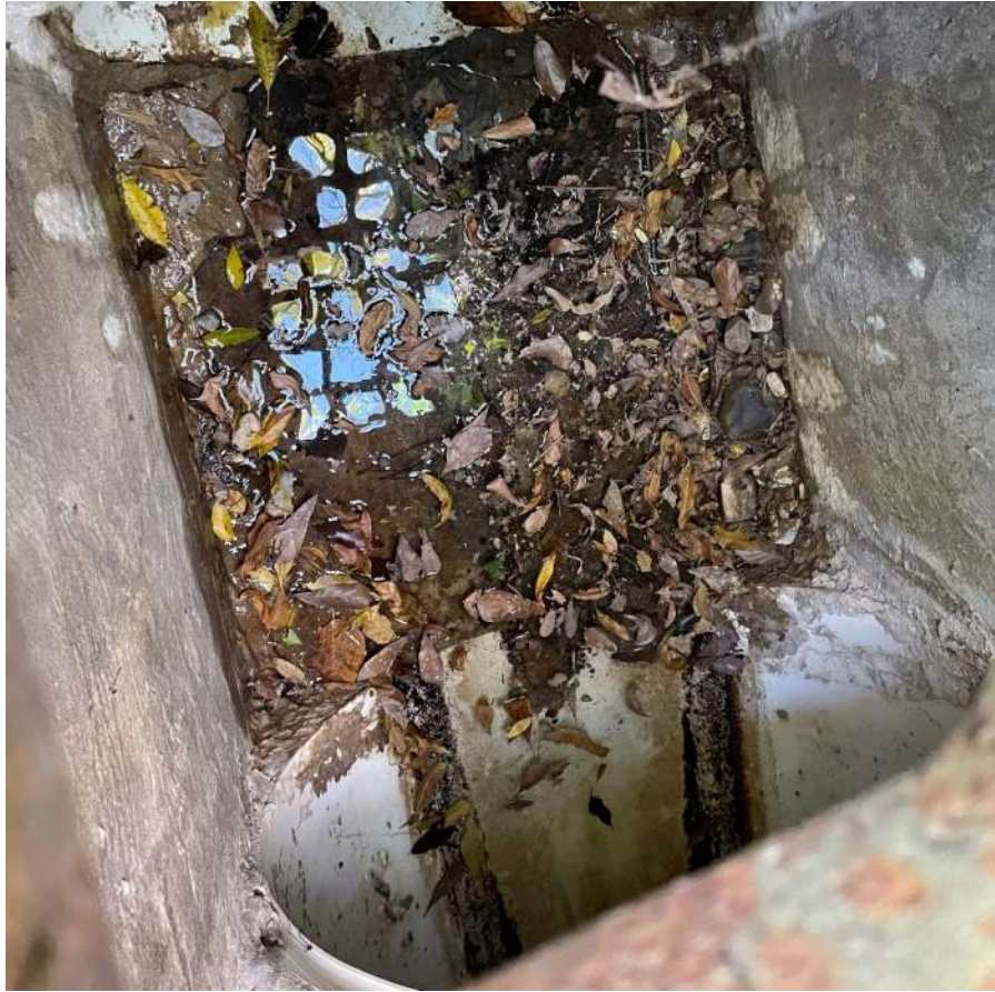
Down View Inlet located on 625 Piney Point Property
