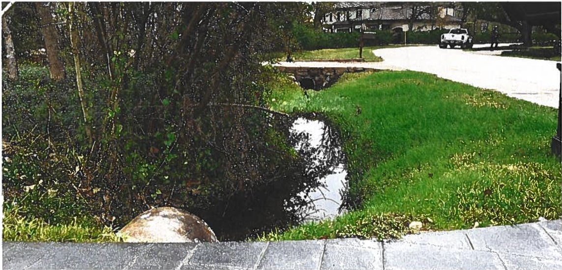
DITCH BETWEEN #6 & #4 LACEWOOD
