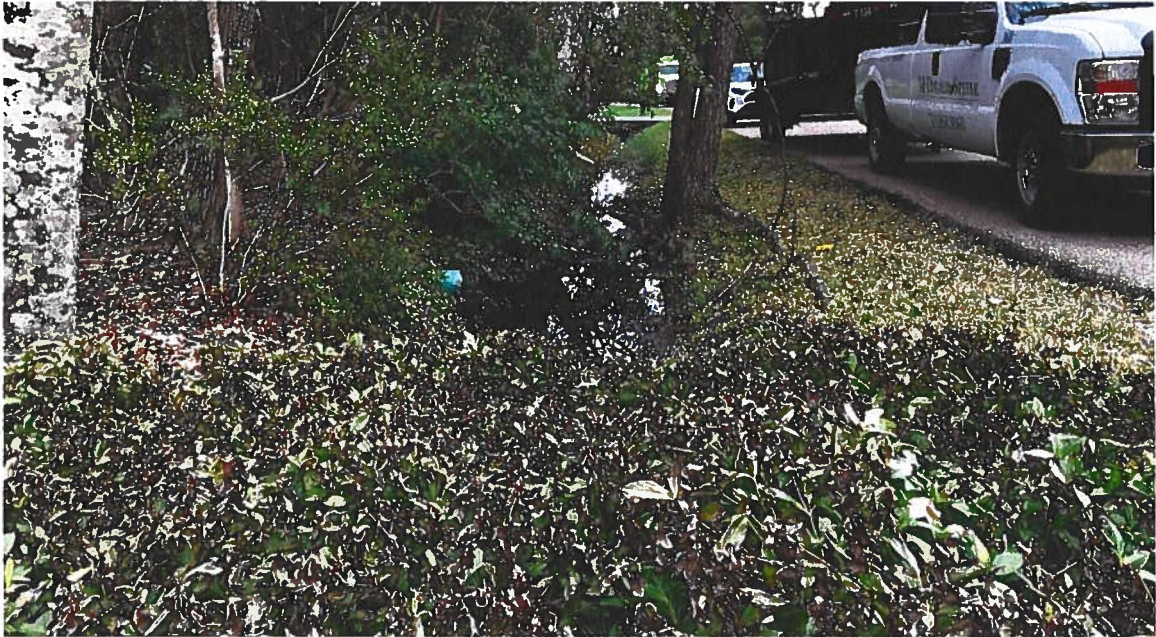
DITCH BETWEEN #8 & #6 LACEWOOD
