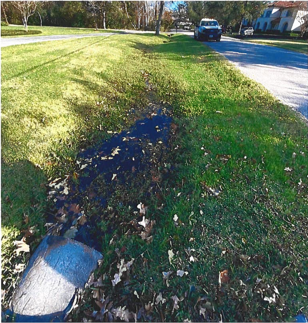
DITCH AT #6 LACEWOOD
